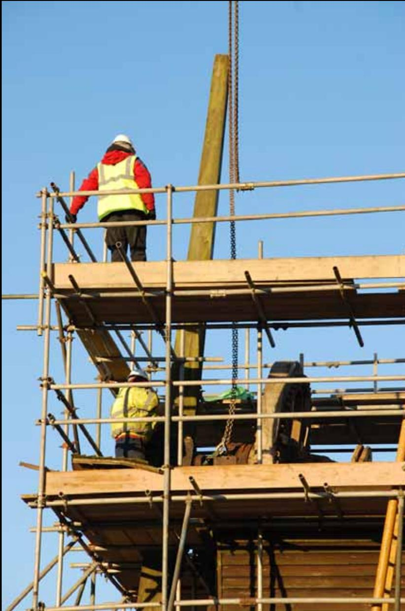
Contractors free-up the remaining sail stock and connect the crane's lifting straps.
