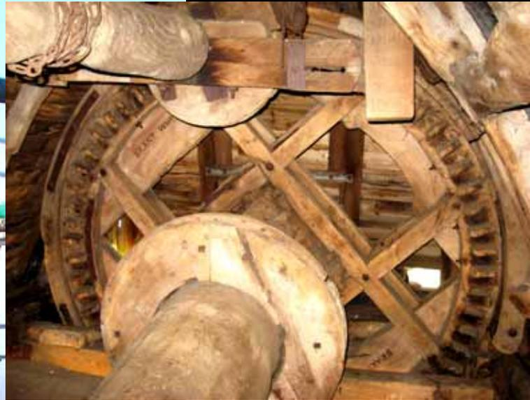
Next for removal is the large brake, brake wheel and shaft which sit at the upper floor (the Bin Floor) of the mill.
