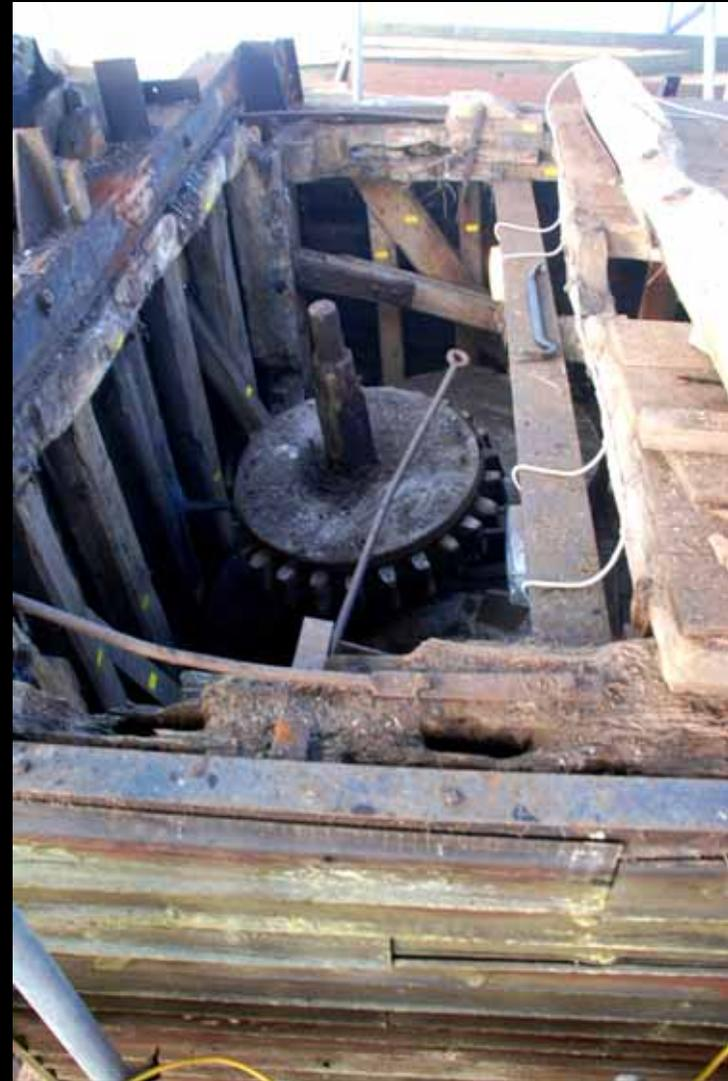
The wallower (gear and shaft in centre of photo) and one of the millstones can be clearly seen. These are next for removal
