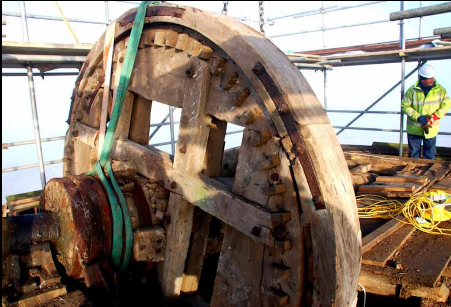
The crane's straps are properly secured on either side of the brake wheel and the last checks are made to ensure that the structure is free for lifting
